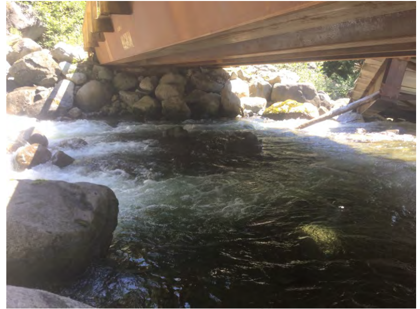
Left Bank Abutment when facing downstream
