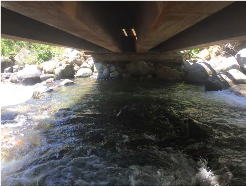
Right Bank Abutment when facing downstream
