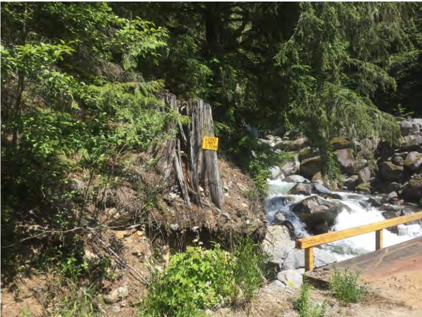
Load Rating Sign
